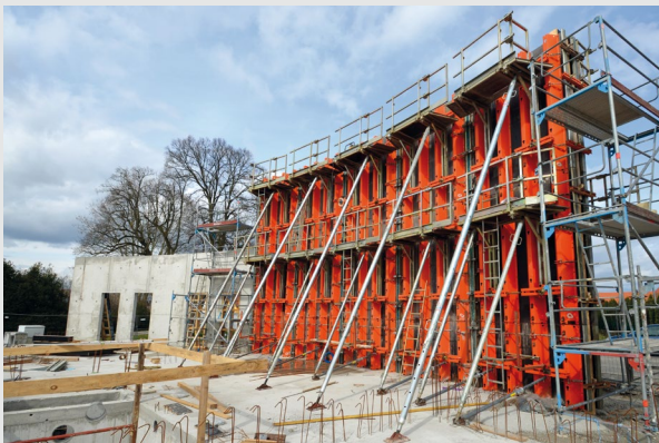
Adjustable prop 400-620 cm on a construction site in Beinheim
