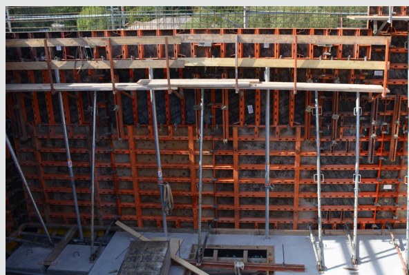
Adjustable prop 255-405 cm on a construction site in Sömmerda
